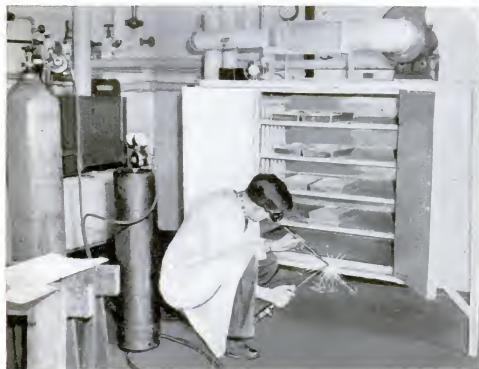
An engineering student puts finishing touches on a laboratory oven drier
